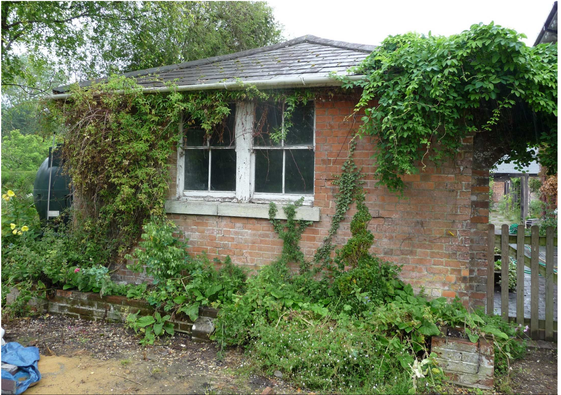
PHOTO - FRONT ELEVATION OF OUTBUILDING
