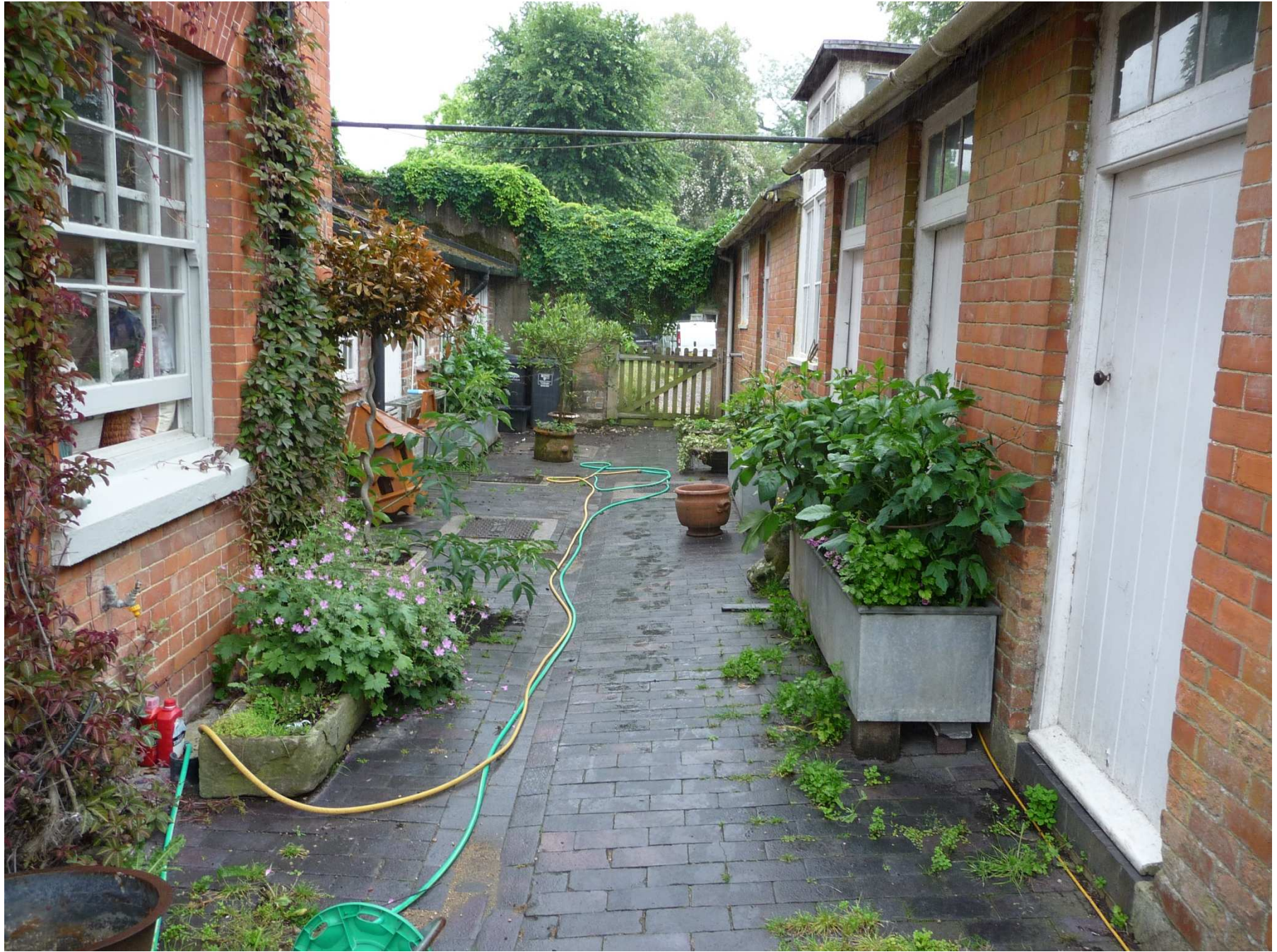
CONNECTING COURTYARD – FACING SOUTH
